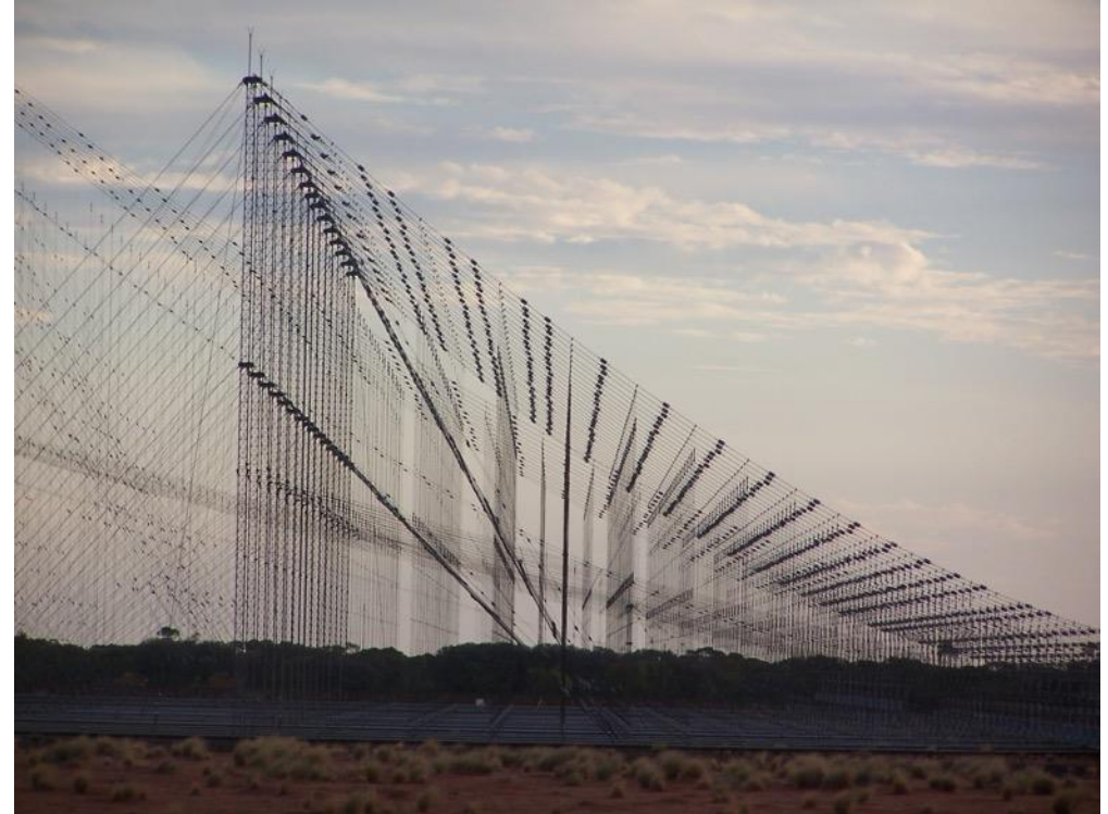
Australian JORN transmit array – Laverton, WA. On transmit vertical log periodic arrays are common.
