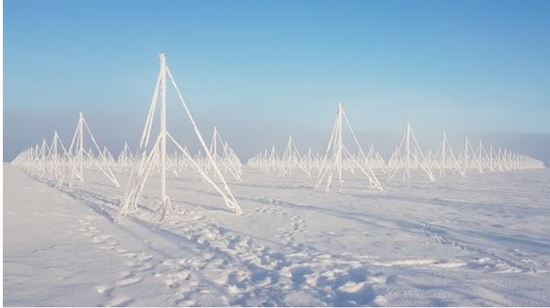
Canadian P-OTHR array, after Riddols (2022). On receive vertical monopoles are common.
